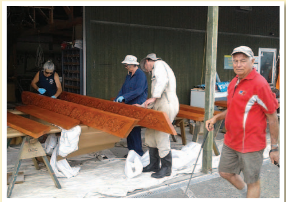
Marae workers brushing on wood conditioner to etched panels.
