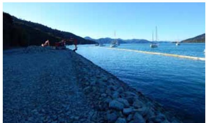
*Rock being placed for new marina. The silt curtain is visible on the right of the image.*
