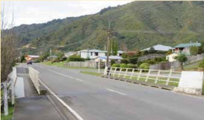
Waikawa Bridge July 2 2019.
