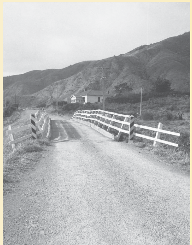
The 1924 bridge in July 1961 before demolition.
